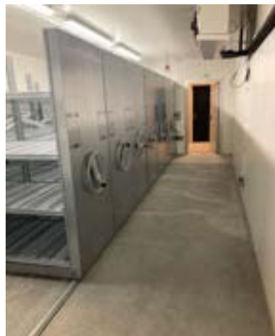
Galvanised fronts, bolted rails
